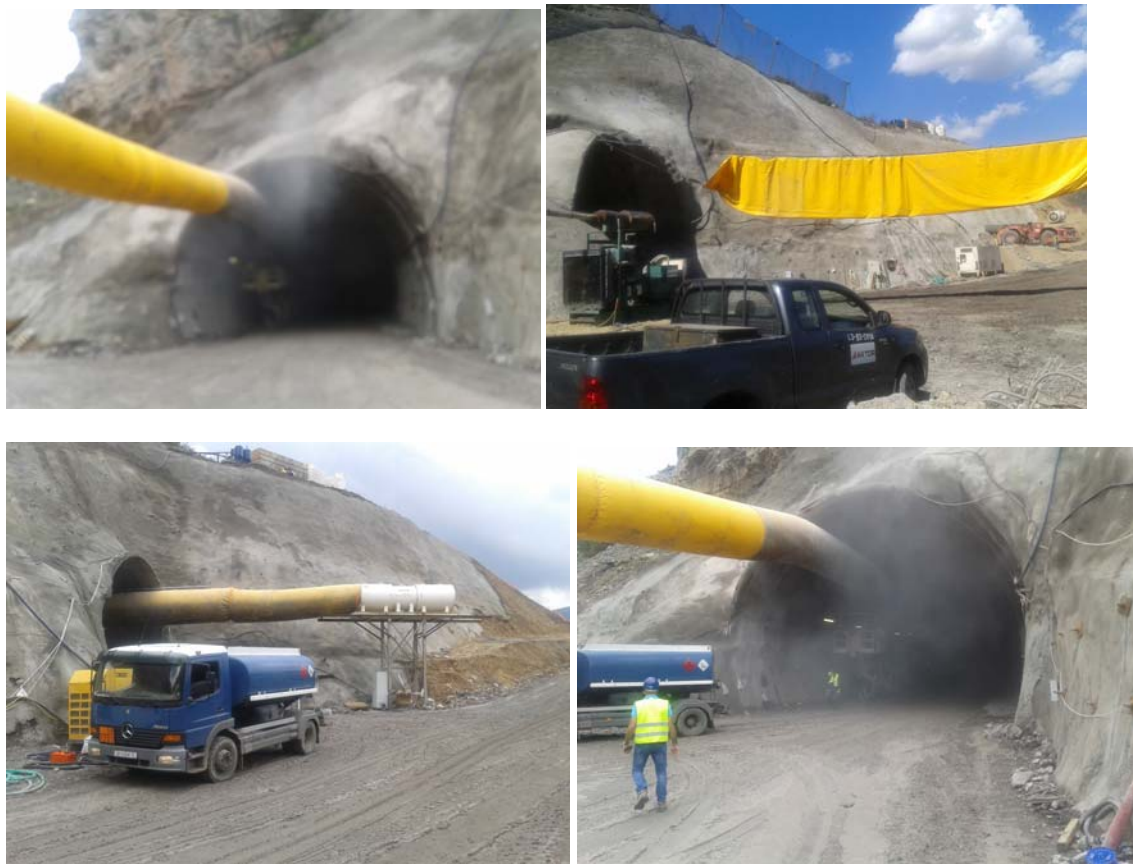
Figure 5. Textile filters (in the tube) remove and filtrate gases from the tunnel
