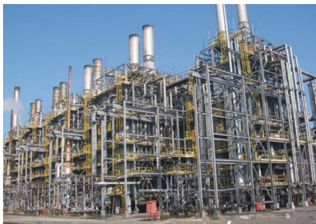
Figure 1. Pyrolysis furnaces in ethylene plant
