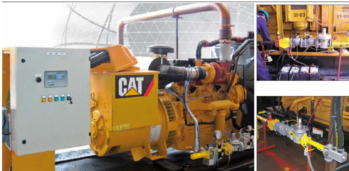
Figure 4. Picture of installed bi-fuel by ComAp on Caterpillar engine C15. (Courtesy of ComAp)
