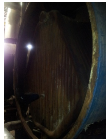
Figure 3. Schematic representation of water-cooled front hot gas reversing chamber (left), the current state of water-cooled pipes (right)
