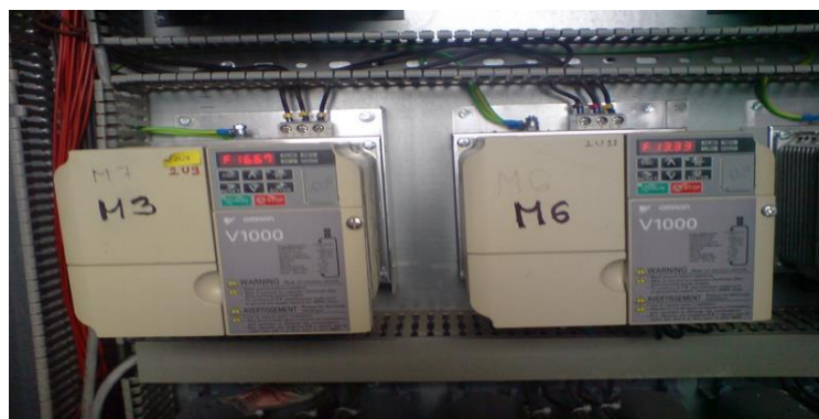
Figure 4. Frequency regulator OMRON V1000
